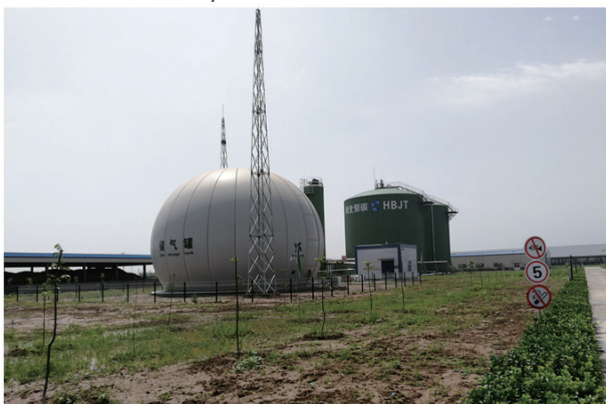
Demonstration Project Site
